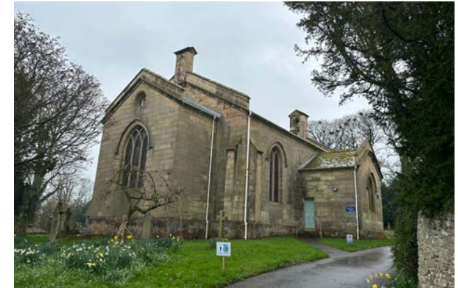
Figure 07: St Peter's Church (Grade II)
