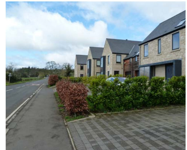
Figure 42: Residential properties in Chollerford, set back from the B6318. These properties have a more contemporary aesthetic to them. Materials and architectural detailing can be found through use of timber cladding and projecting bays powder coated aluminium. Small garden frontages with hedgerow boundary reflect the rural character.
