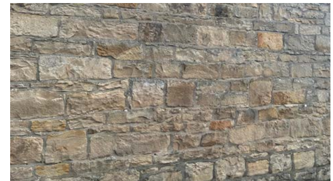
Figure 52: One example of sand stone coursing.
