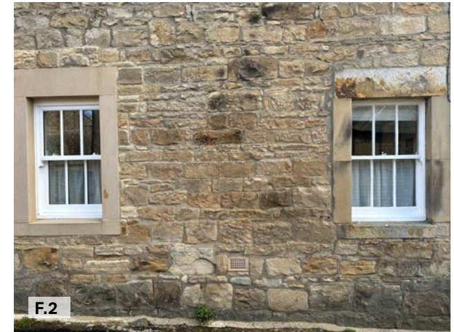
Figure 54: Sympathetically converted windows on a property within Humshaugh Village
