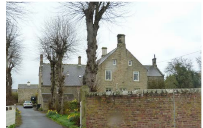
Figure 08: Property within Conservation Area (Grade II)
