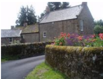
East Farm and Cottage with lichen covered boundary walls
